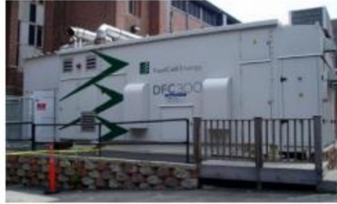
FuelCell Energy – 300 kW MCFC – Connecticut, USA
