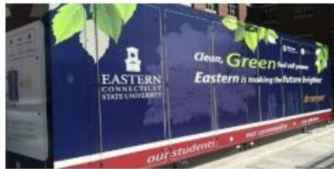
UTC – 400 kW PAFC –Connecticut, USA
